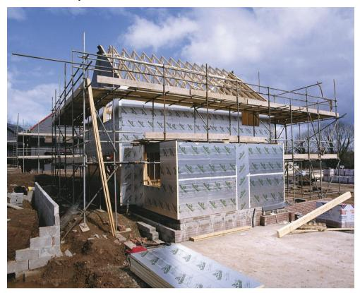
Kingspan Thermawall TW55 and Kooltherm K12 Framing Board are currently the only insulation products compliant to Category B of the criteria set by the Health & Safety Executive (HSE) and the UK Timber Frame Association (UKTFA).
